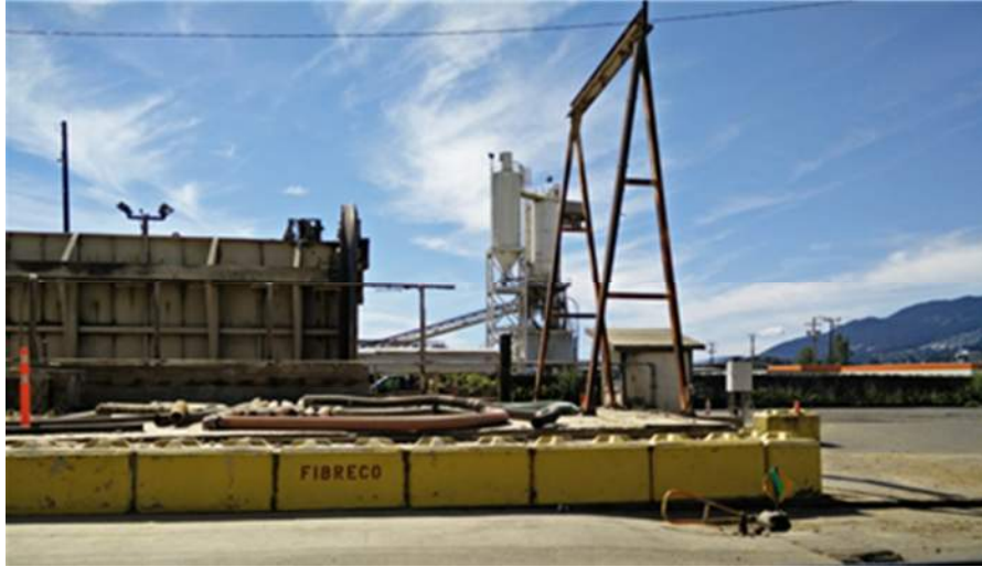
Figure 1: Existing Laydown to be Demolished, Looking West
